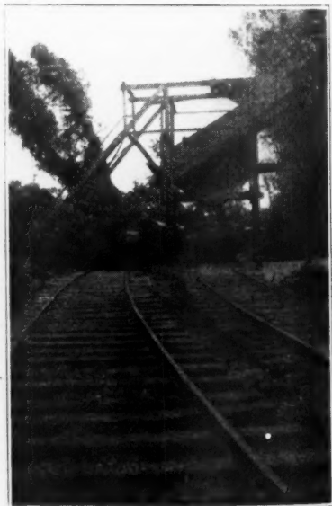
The Track to the Loading Bin
